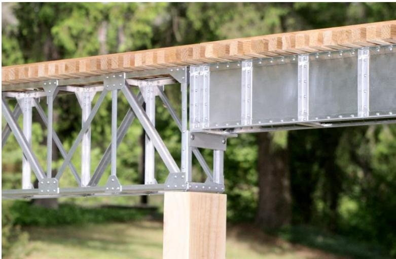
A feature that we wanted was real rivets; the real blood, sweat and tears kind of rivets that my grandfather made in Scott's shipyard in Greenock in Scotland, so special tools had to be bought or designed and made to do this. A basic requirement was that all materials must survive outdoors in all climates, and we think we've got that right. Most structural parts are aluminium alloy, threaded
